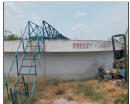
ETP system for water recovery
