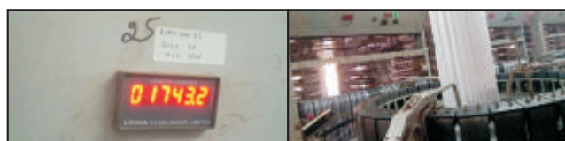
Old Equipment without Machine Controller
