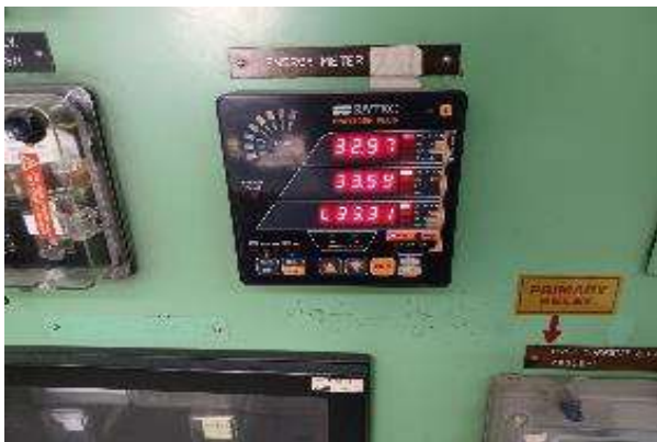
Verifying energy metering system at Chakmir 132kV Substation & Power Transformer at outdoor
