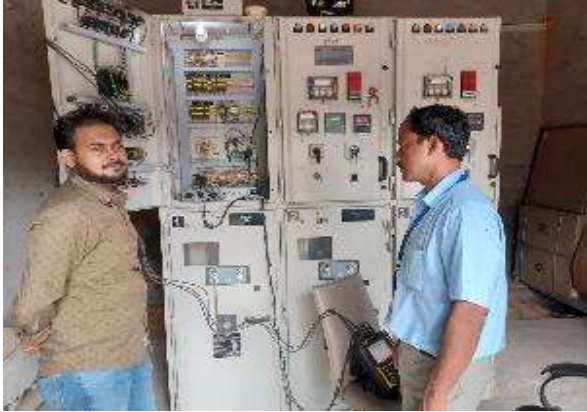
Load Flow & Overloading Checking at 11 KV VCB HT Supply Point of Ruby General Hospital
