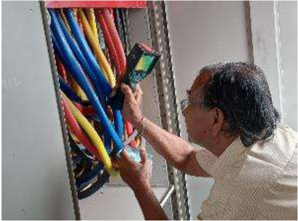
Thermal Imaging carried out by AEA at Incomer of LT PCC Panel of Ruby General Hospital
